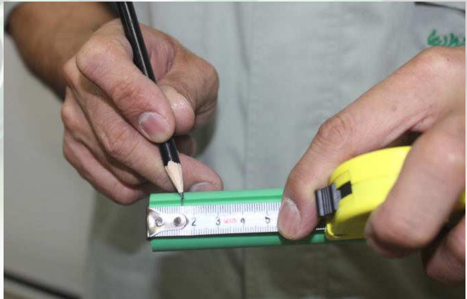
Fig. 11: PPr-FG Pipe Socket Depth Marking
