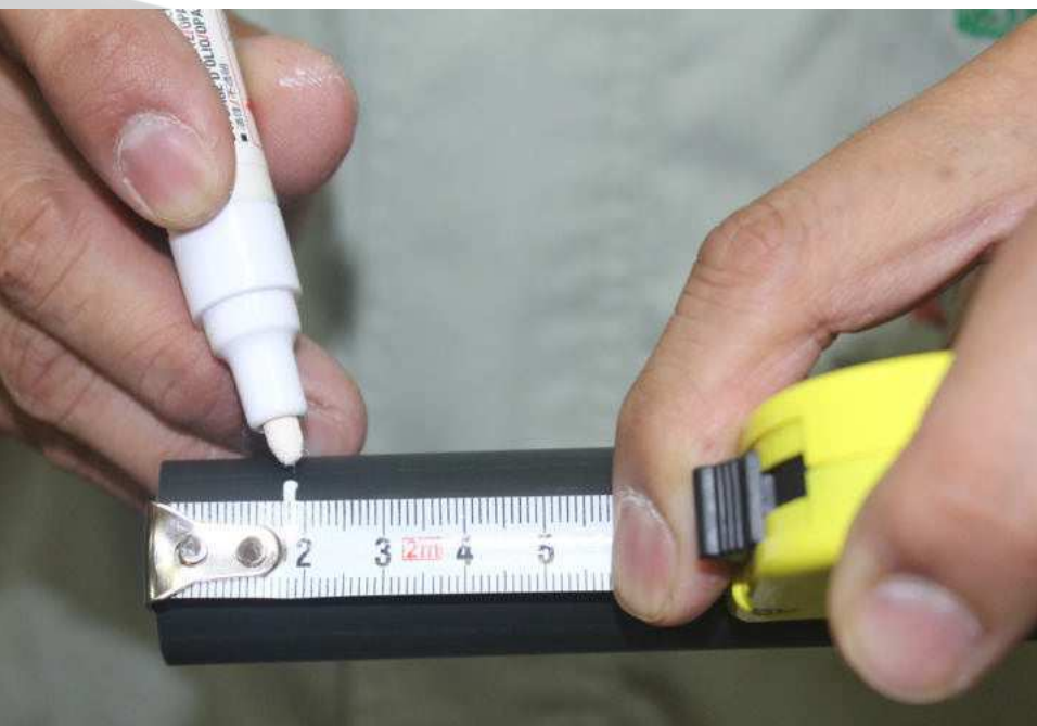
Fig. 10: PPr-PE Pipe & PPr-FG-PPr-PE Pipes Socket Depth Marking
