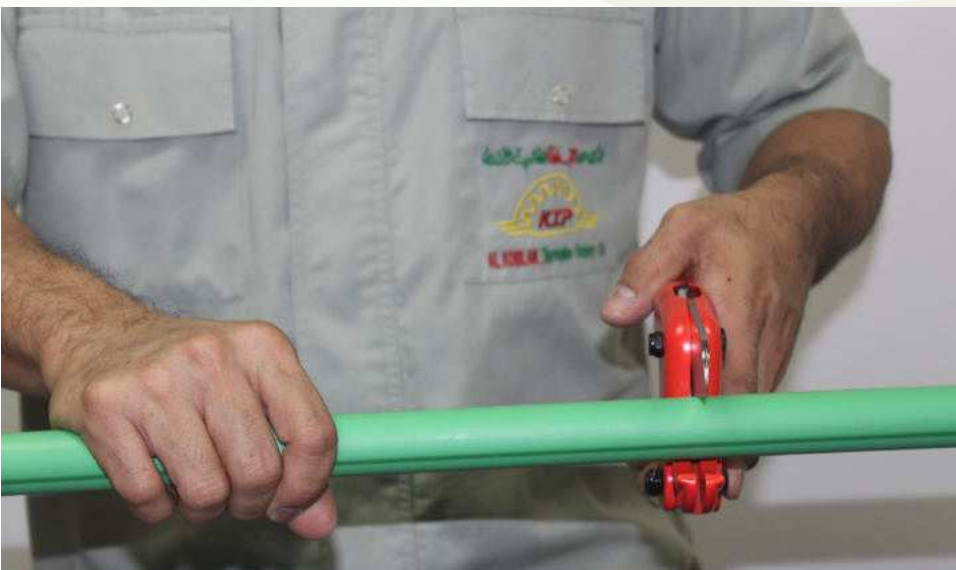
Fig. 9: PPr-FG-PPr Pipe Cutting
